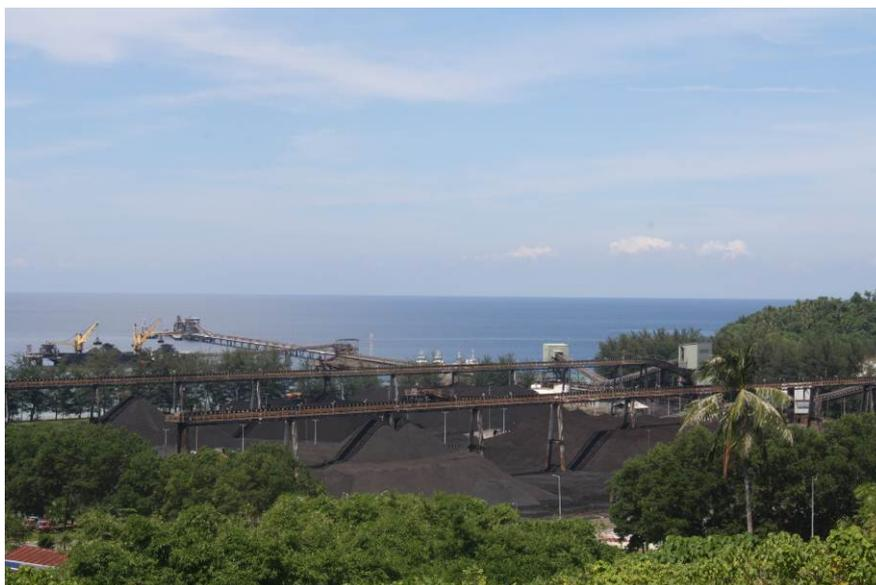
*IBT has eight stockpiles with total capacity of 800,000 tonnes and has two conveyors to blend two types of coal at a given time*
